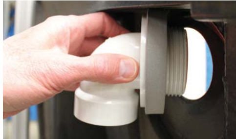
Overflow ell extends through hole
